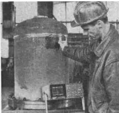
Fig. 28.5. Manual weld testing in chemical plant construction with digitized miniature, flaw detector USD 10 (design Krautkrämer)
